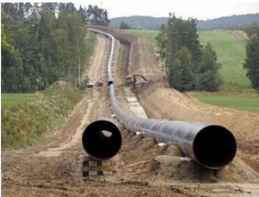
Figure 4: Pipeline construction in Western Bohemia
