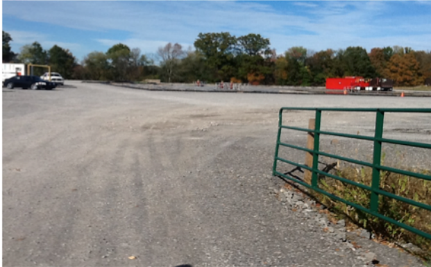
Figure 4 - Well site under construction showing banded area.
